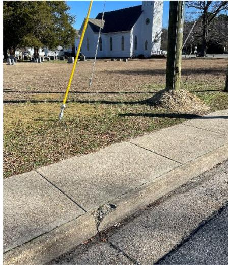
Item 2: Slab on King Carter Drive next to manhole in front of Steamboat Era Museum is shifting and cracking (New)
