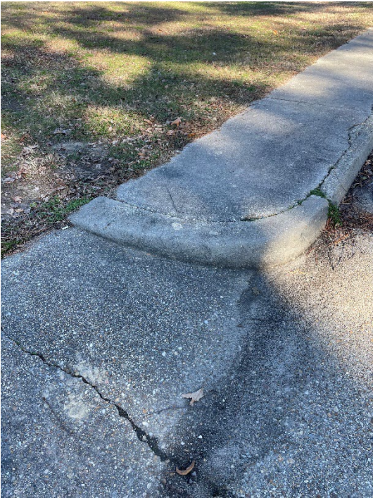
Examples of sidewalks which cannot be navigated by wheelchairs or mobility scooters, mostly on driveway cuts on Irvington Road and Steamboat Road
