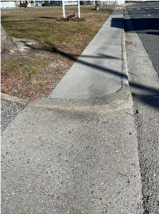
Examples of sidewalks which cannot be navigated by wheelchairs or mobility scooters, mostly on driveway cuts on Irvington Road and Steamboat Road
